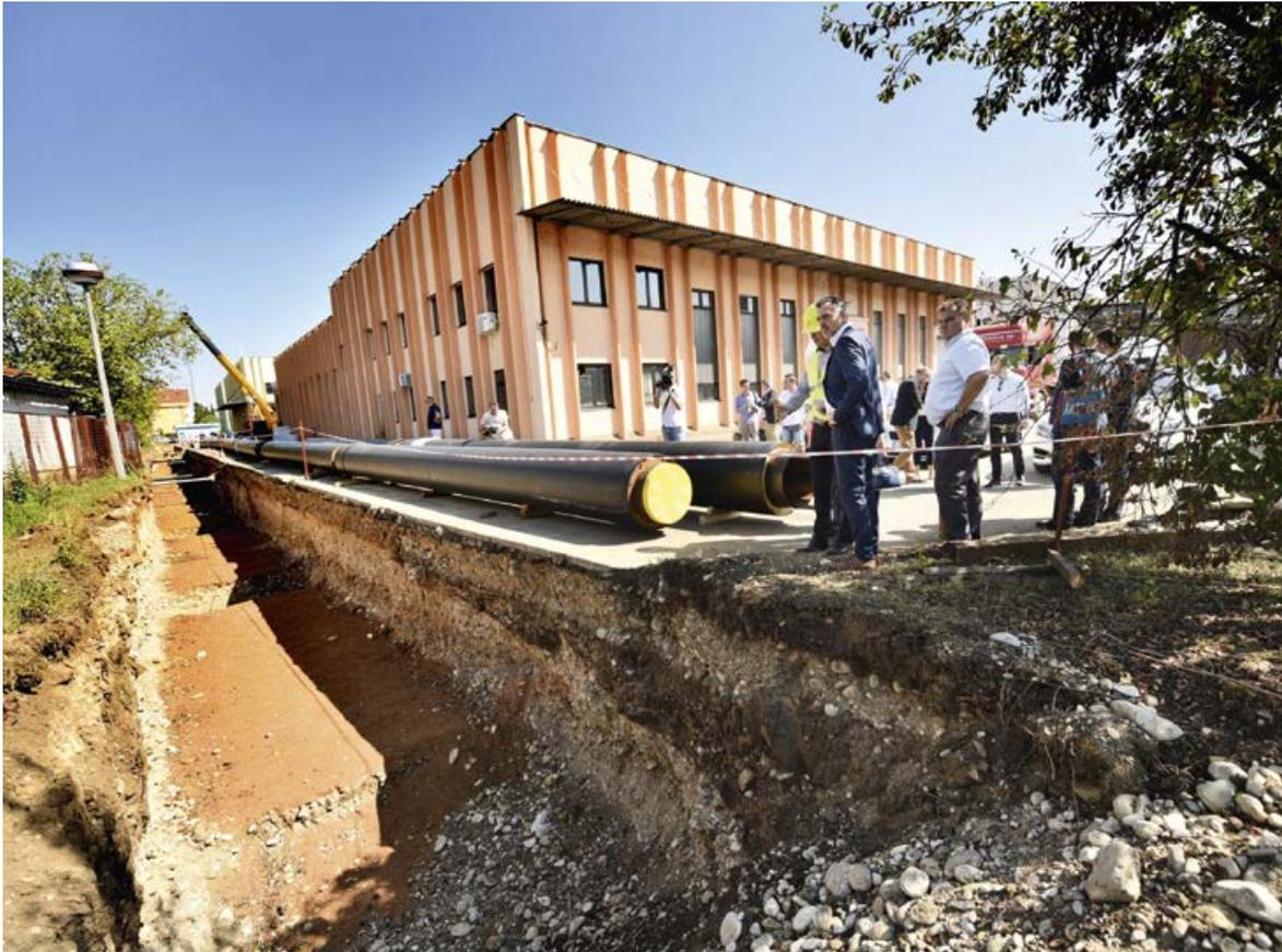
Pipes being laid during the construction phase of the new Banja Luka district energy system.
