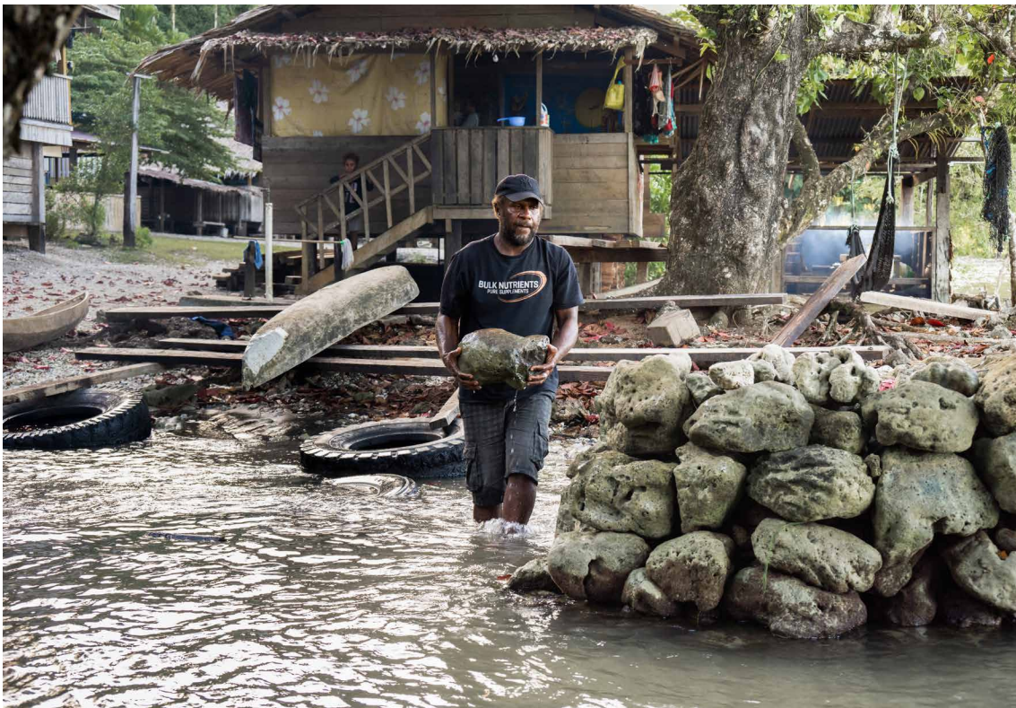
Martin Hau'ato collecting rocks for his community's sea wall that stretches across the shorelines of Muki Community in the Solomon Islands. The creation of the sea wall is made up of coral stones collected from deeper in the ocean, and brought to shore using small dugout canoes. Photo: Ivan Utahenua/Oxfam
