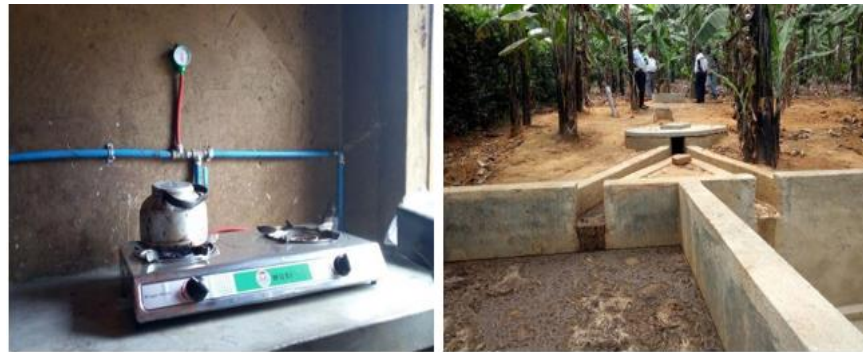
Figure 3.22: Biogas for cooking at household level in Rubirizi District, and Bio-digester plus Bio-slurry in Mbarara District, both offering mitigation co-benefits.
