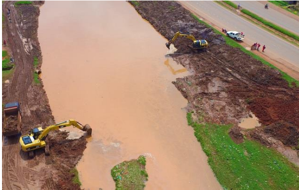
Figure 3.32: KCCA expansion works of Lubigi, Nakamiro drainage channels
