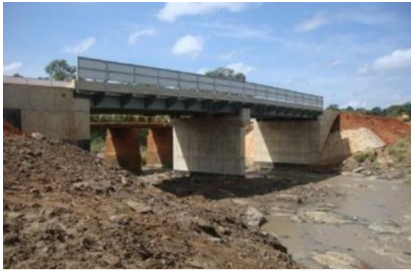
Figure 3.30: Climate proofing road infrastructure: construction of Moyo Nyawa Bridge
