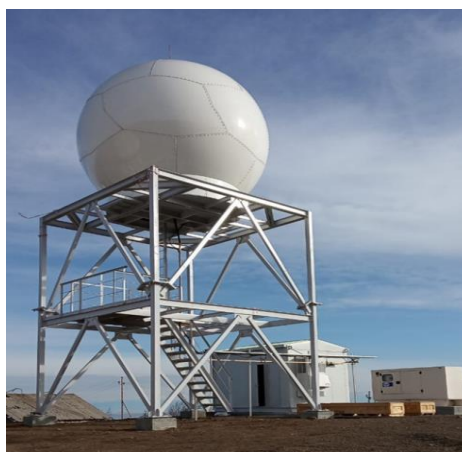
Figure 4-22. Modern Doppler radars installed in Goygol and Shamakhi districts
