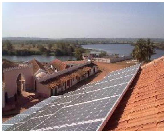
Bambadinca Solar Plant - Guinea Bissau http://suniaenergy.com/trabajos/central-solar-de-bambadinca-guinea-bissau/
