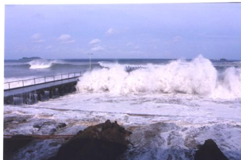
Photo 1: Hurricane Lenny Storm Surge
