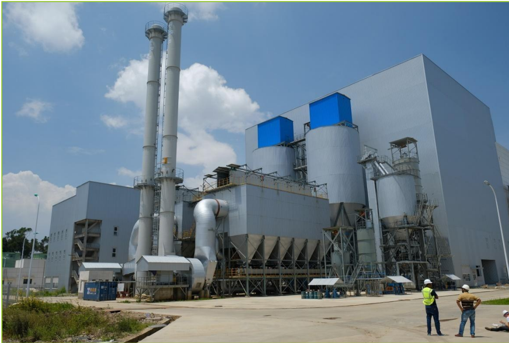
Figure 99 Reppie Waste-to-Energy facility
