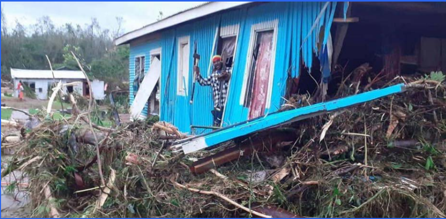
A destroyed house in the Fiji village of Cogeia.
