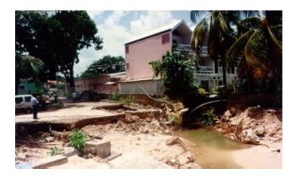
Figure 2.2: Erosion at Holetown, St. James.
