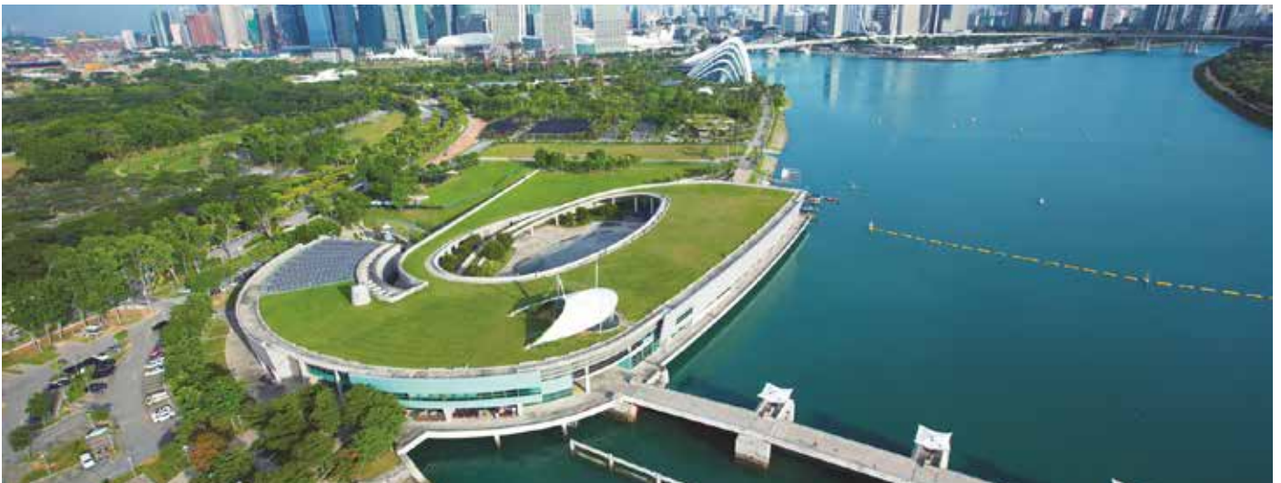
More than just an ordinary dam, the Marina Barrage serves three benefits: it creates a freshwater reservoir to boost Singapore's water supply, acts as a tidal barrier to prevent flooding in the low-lying areas in the city and offers a venue for water-based recreation.
