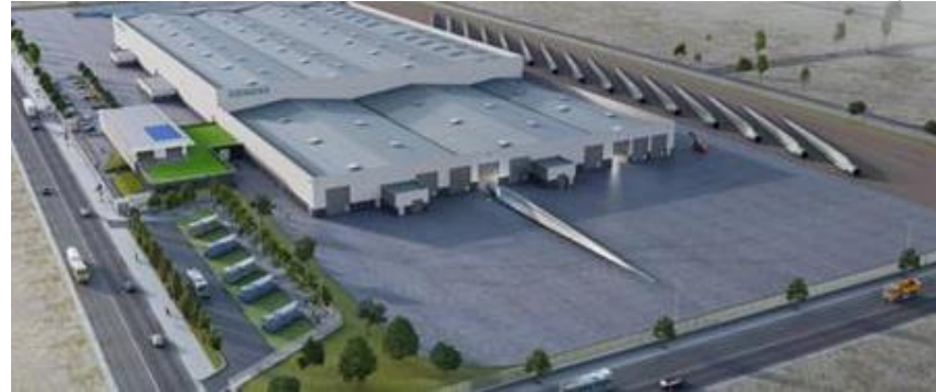
manufacturing of wind turbine pallets (Tangier Factory)
