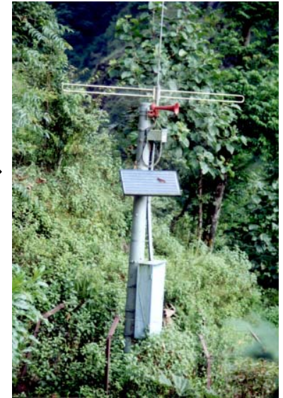
GLOF Warning System
