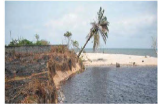
Erosion at Sablière
