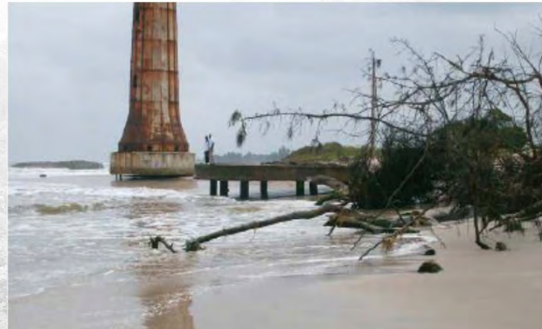
Erosion at Cap Lopez
