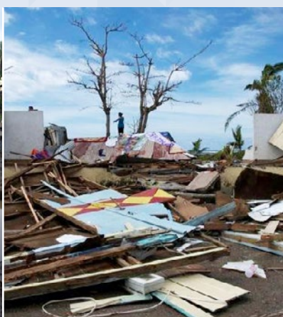
Damage from Cyclone Evan, Samoa 2010
