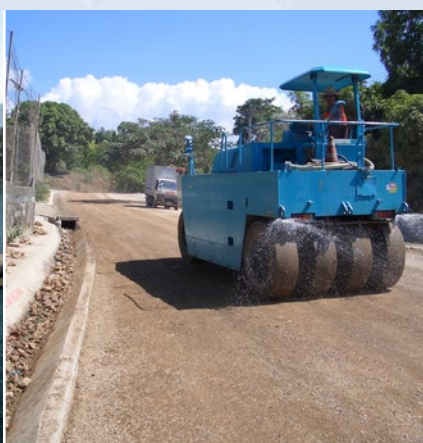
Roading upgrade, Solomon Islands
