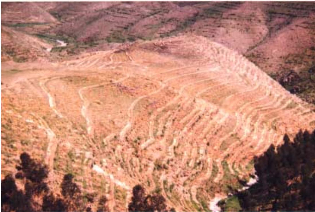
**Figure 4.1: Typical example of terracing for soil and water conservation and tree planting activities.**
