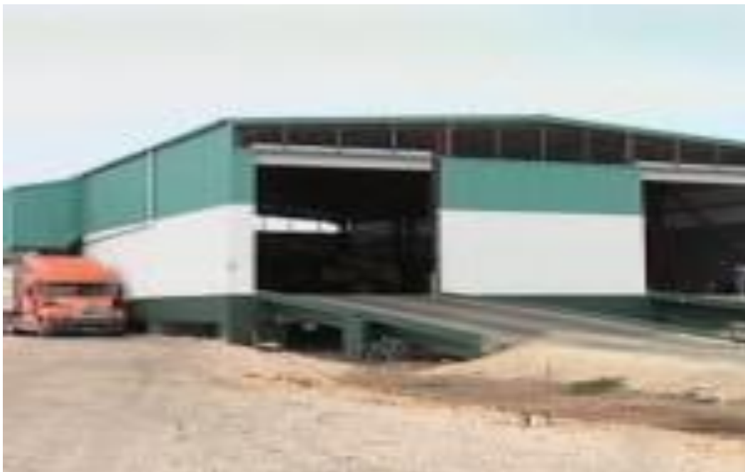
Figure 52: Transfer Station located at mile 3, Gorge Price Highway (Inaugurated 6 th August 2013) Source: Great Belize Productions Limited
