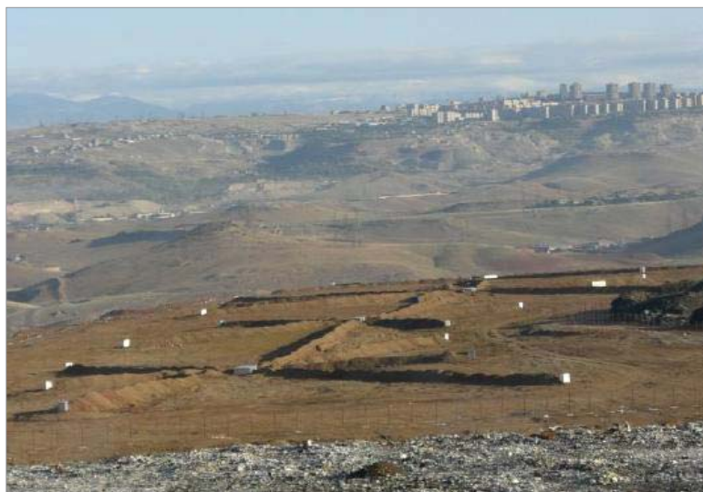
Figure 4.4.3 “Nubarashen” SWDS: Location of Methane Capture Holes, Yerevan
