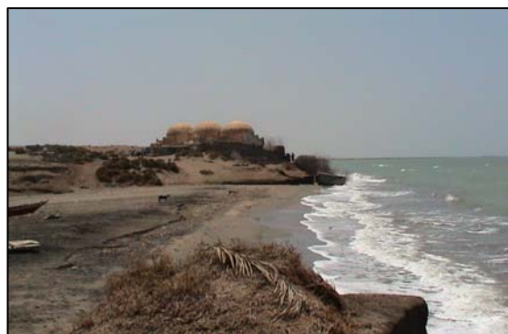
Figure 3-2: Coastal erosion, Alfazaa Mosque
