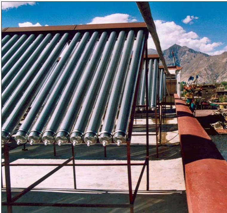
Figure 1: Evacuated Tube Solar Collector in Tibet, China.
