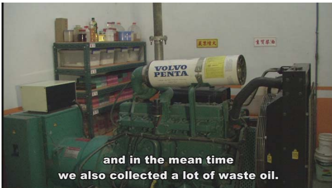
5. Make bio diesel fuels for Community's emergency generator.
