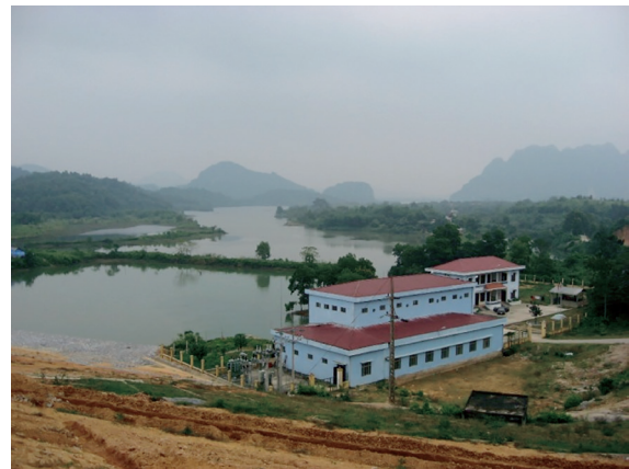
Small hydropower plant in Muc River, Thanh Hoa Province
