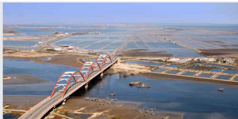
Bird's-eye view of the SSTECH in 2008. The original site comprised non-arable saline land and polluted water bodies.
