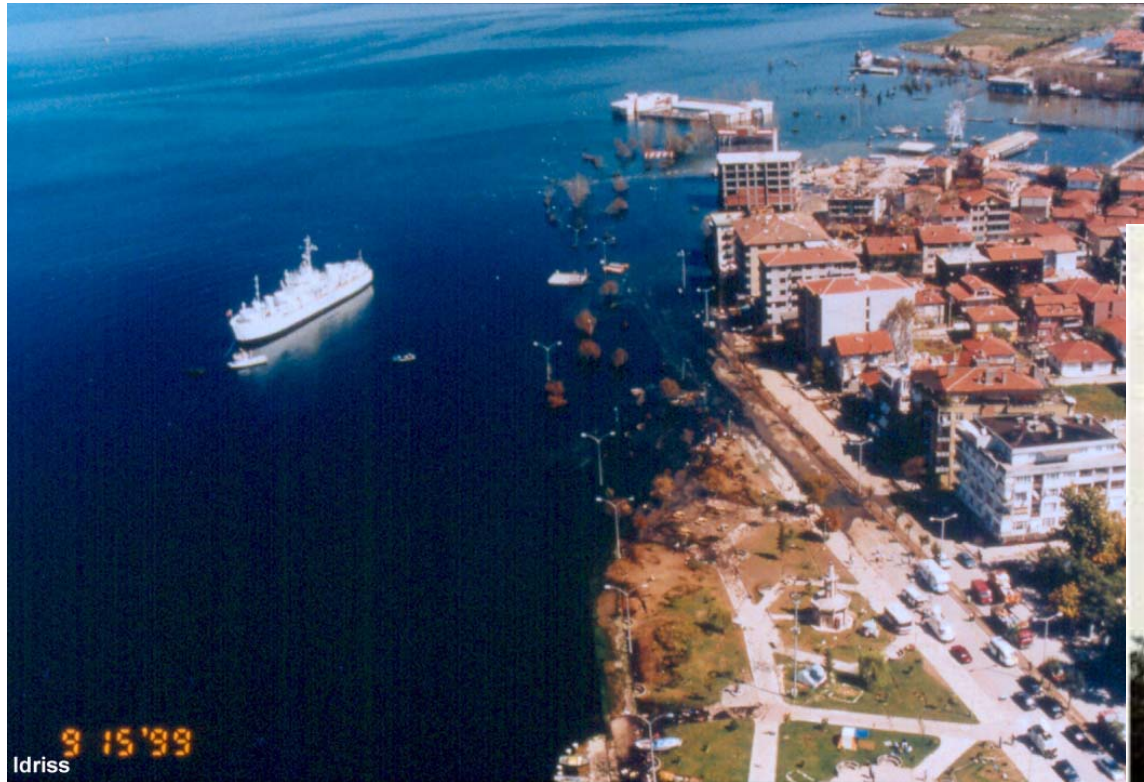
Sudden subsidence on the coast of Turkey following an earthquake in 1999
