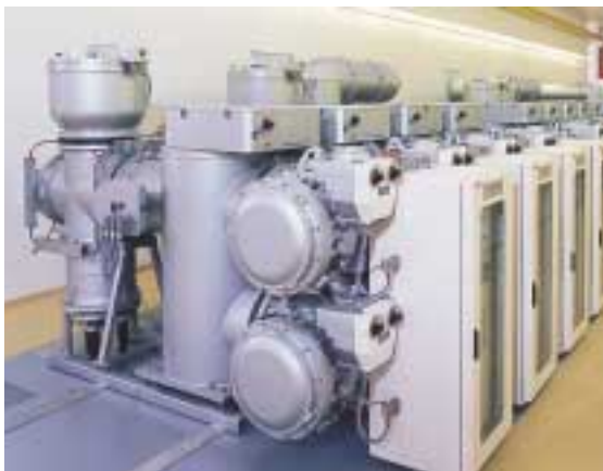
In gas-insulated, metal-enclosed high-voltage switchgear, SF 6 is used as an insulating and arc-quenching medium.
