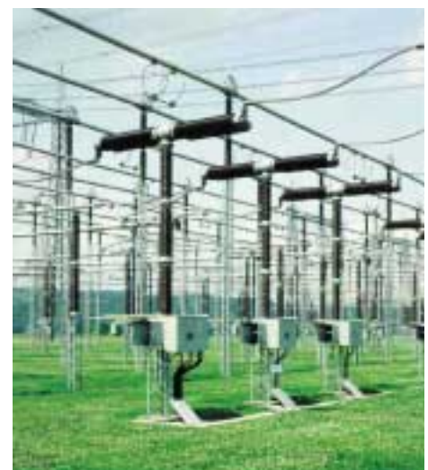
Outdoor-type transformer substation with SF 6 equipment
