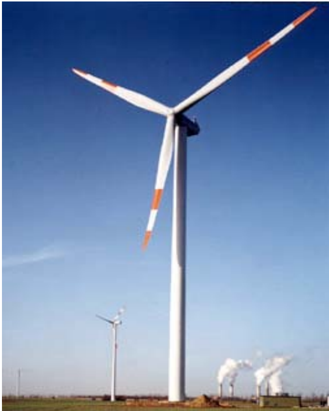
Prototype of 80 m tall Nordex 2,5 MW wind turbine located in Grevenbroich, Germany (Danish Wind Industry Association)
