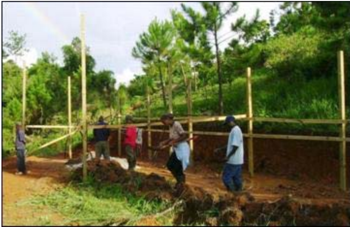
A community in Jamaica working on slope protection against erosion
