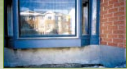
Foundation wall cracks (North-facing windows reflect seniors' housing development on former church property).
