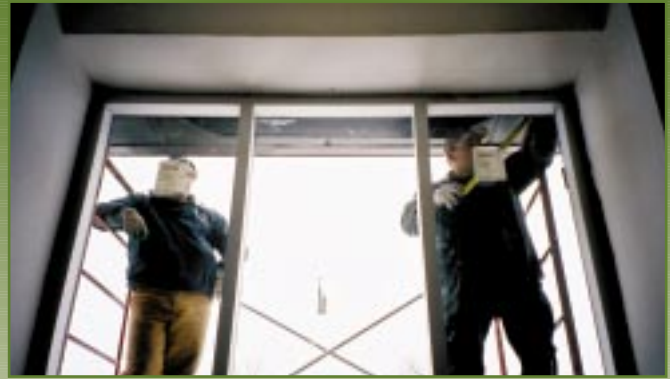
Interior view of new windows installation.
