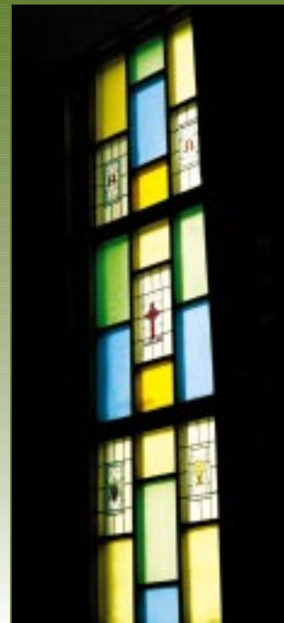
Stained glass windows — beautiful, but a special energy-efficiency challenge. Caulking, weather-stripping and exterior mylar protective shields cut down heat loss without affecting light.
