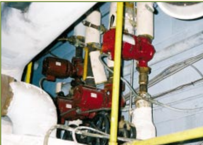
Complicated old boiler system.
