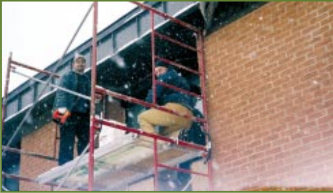
Exterior view of new windows installation.
