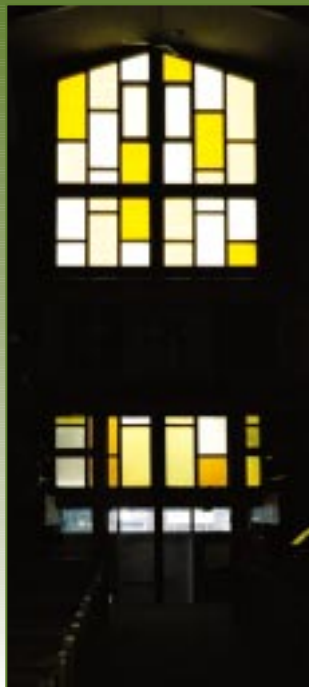
Sealing the south door and stained glass in rear church wall reduces heat loss.
