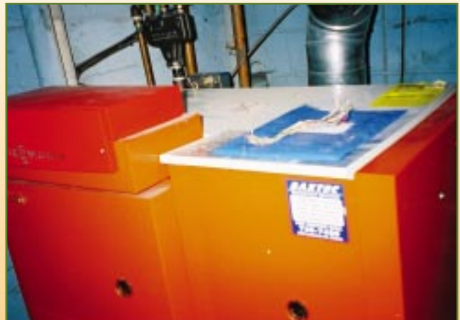
New high energy efficient boiler.
