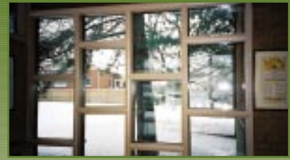
Re-caulking of many windows and doors in the link area improved building envelope integrity.
