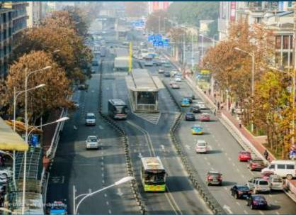
**Yichang BRT** Unique Station design for narrow road and medium scale cities, and first automatic BRT boarding platform in the world
