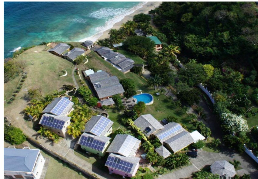
PV System atop Maca Bana Villas and Aquarium Restaurant, Grenada (Photo credit: Maca Bana Villas and Aquarium Restaurant)
