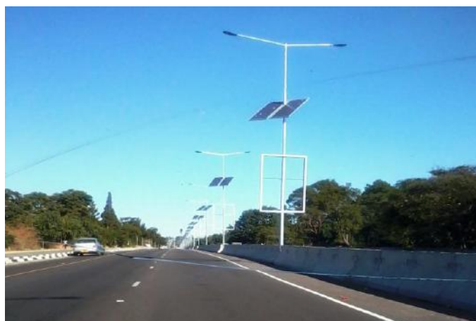
Figure 4. Street solar lighting project in Harare
