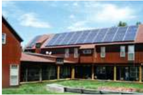
Solar Home System for lighting
