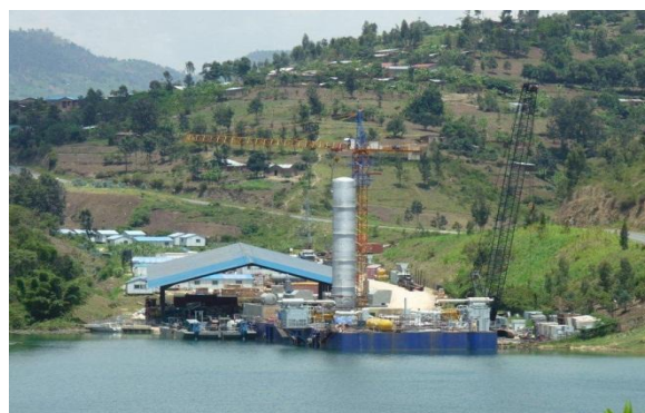
Picture 8: Lake Kivu 25MW methane gas power station in Rwanda
