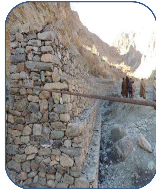
Protection Wall at Shogram
