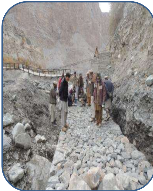
Physical work in Progress in Shogram
