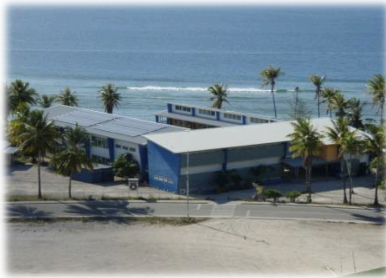
Figure 1: REP – 5 Program PV system at Nauru College (South roof)
