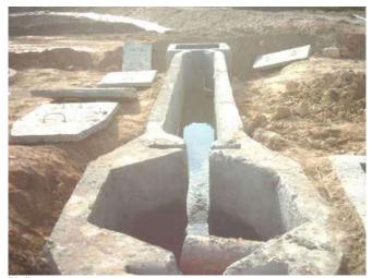
Biodigestor - wastewater treatment
