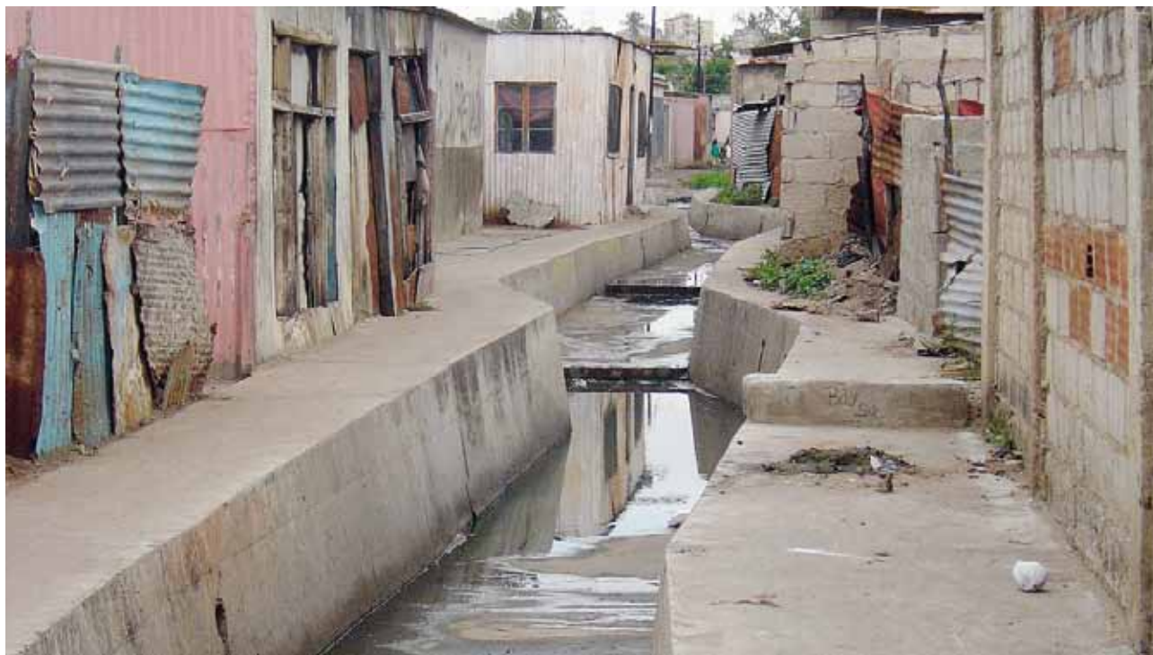
Improved drainage in Mafalala, Maputo ©UN-HABITAT/B.Oballa
