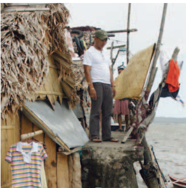
Informal settlements are regularly rebuilt after storm surges that breach the seawalls
