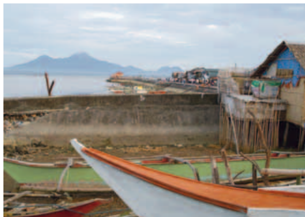
Seawall facing Sorsogon Bay @UN-HABITAT/Bernhard Barth
