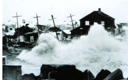
Flood from Storm Surge
