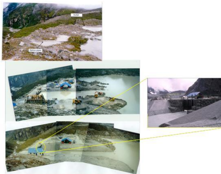
Figure 1: Top picture shows the end moraine before construction. The middle picture shows the site during construction and the bottom picture show after lake lowering. The picture in the right shows details of the control structure.
