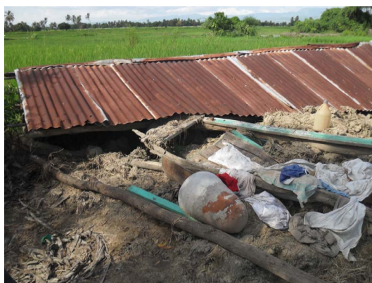
House completely collapsed by rain and winds Source: Fonkoze
