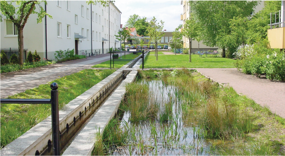
Sustainable urban drainage systems: Suburban regeneration including ditches, retention ponds, green roofs and green spaces has increased climate resilience in Malmö, Sweden, through decreasing rainwater runoff even in heavy rainfall events, and increasing green space, ecosystem services and community spirit
