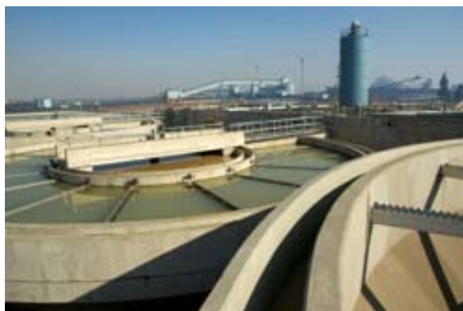
eMalahleni Water Reclamation Plant
