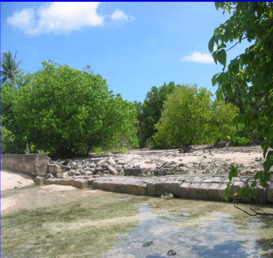
Seawall collapsed
