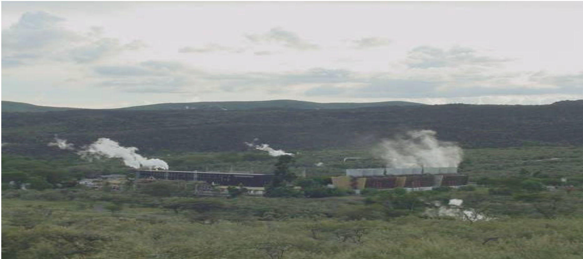
Fig. 2 View of Olkaria I Power Plant
