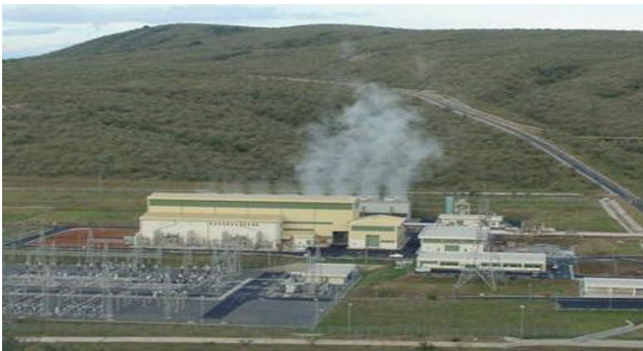
Fig. 3 View of Olkaria II Power Plant
