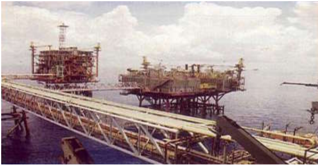
Bach Ho oil exploitation
