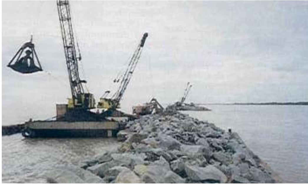
Sea Dyke embankment
