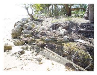
**Plate 4.9:** The seawalls at Manuka, where it has been breached by recent tidal waves, exposing coastal tree roots and ultimately brought it down at places. (Picture taken in early 2003)
