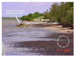
Landward migration of the shoreline is also presumed from fieldwork observations, indicated by fallen trees and exposed tree roots on the shoreline. Remains of possibly an old protection seawall built before 1976 stands 10 - 12meters seaward from the present shoreline also indicate recession of the land (**Plate 4.8**).
