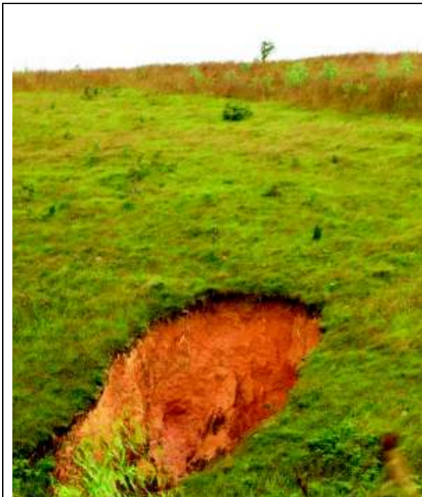
A sinkhole in grassland below recently planted eucalyptus trees. Idete, Tanzania 2010.
