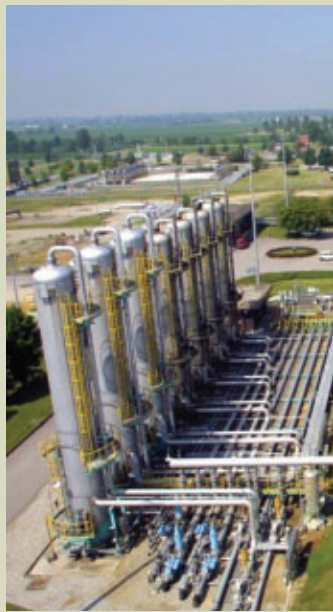
Figure 3.14: Gas storage plant.
