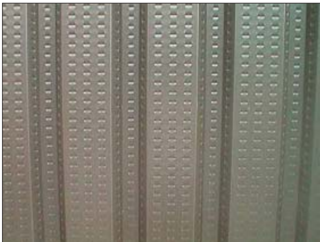
Figure 4: Transpired-Plate Solar Collector.
