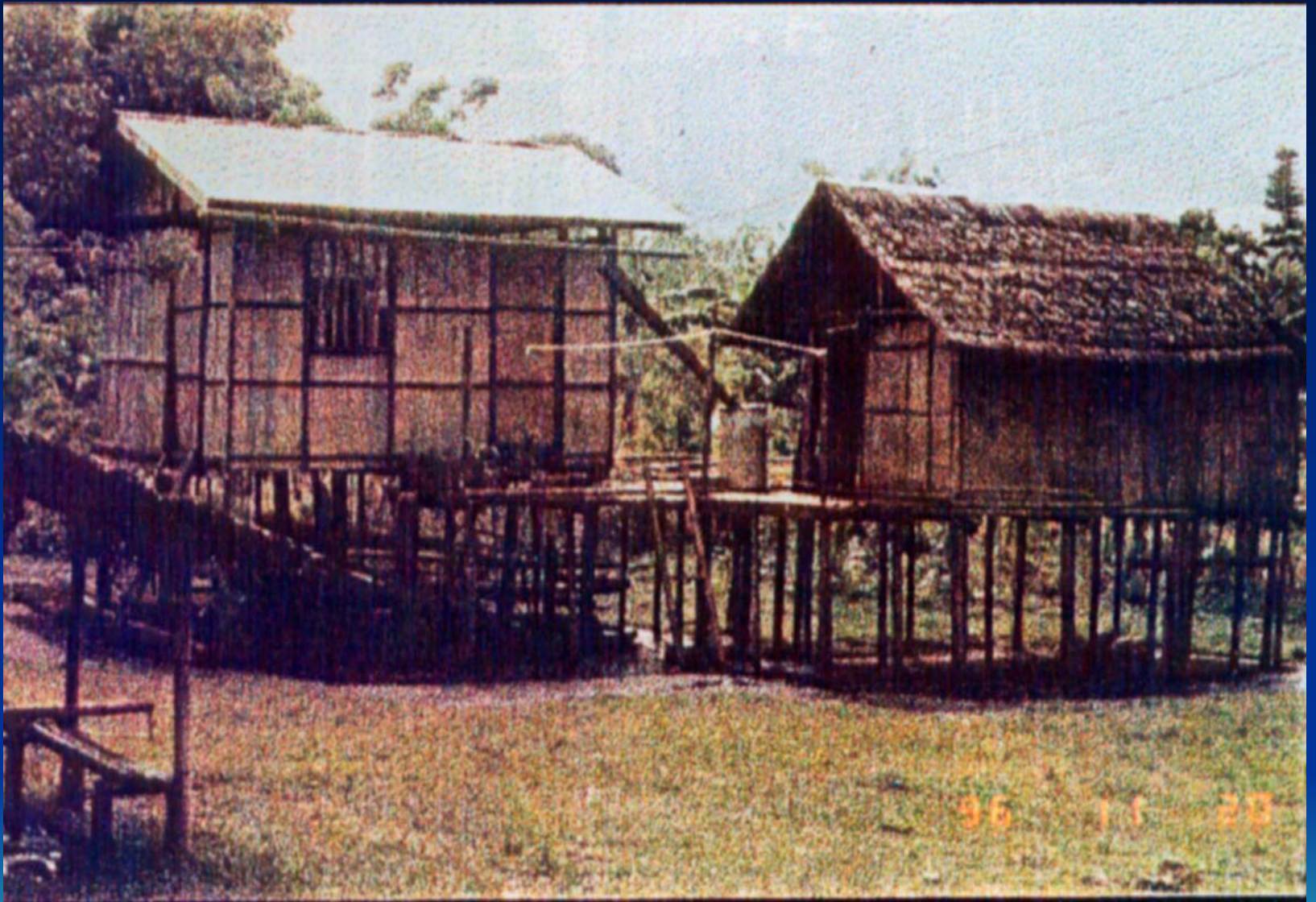
Tausug house with rainwater collection system
